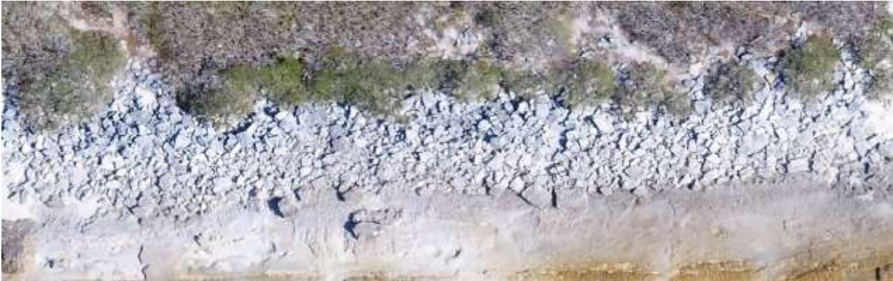
Figure 113. Approximately 80m of lithified shoreline on the southern and windward side of North East Cay. Credit: Graham Hemson ©, Queensland Government
