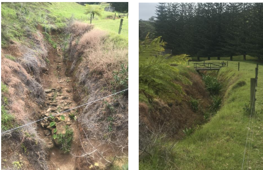
Figure 6: Erosion in Watermill Creek (Wilson, 2020).
